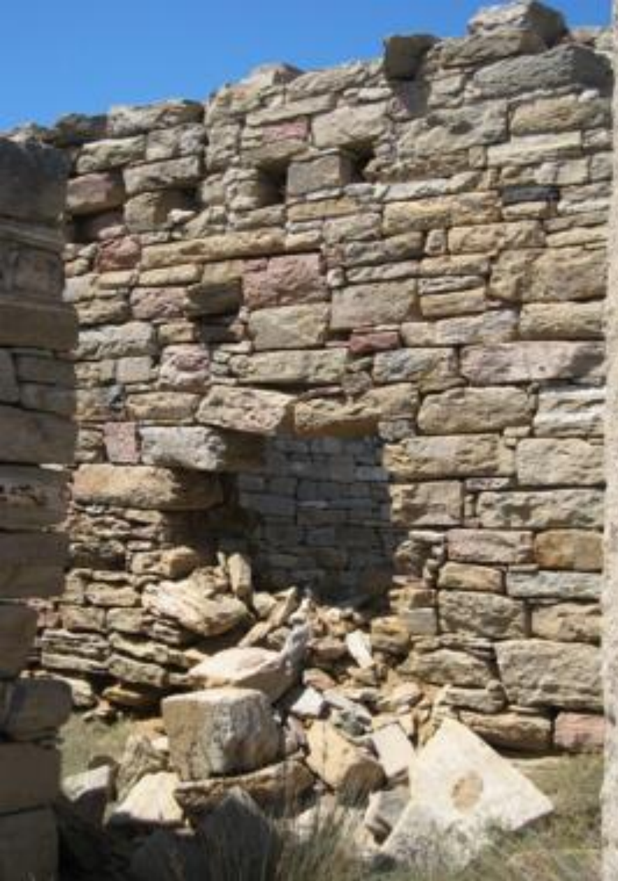
Delos: deterioration of the walls
