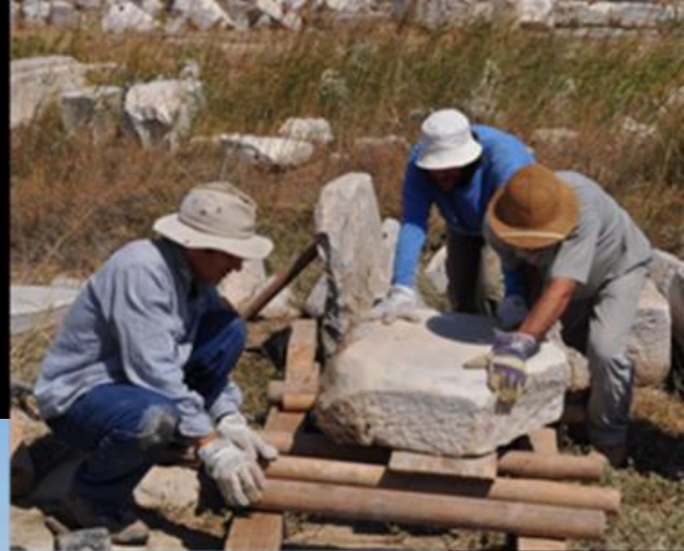
Construction of elevated platforms
