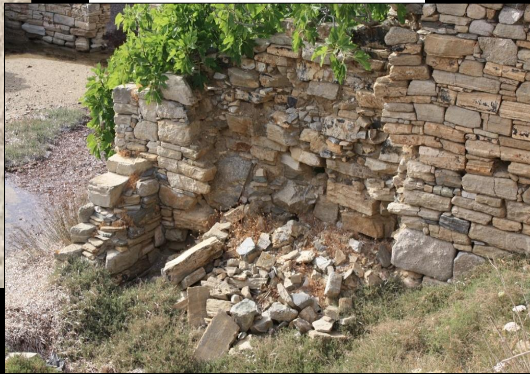
Delos: deterioration of the walls
