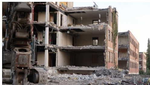
Demolition of buildings
